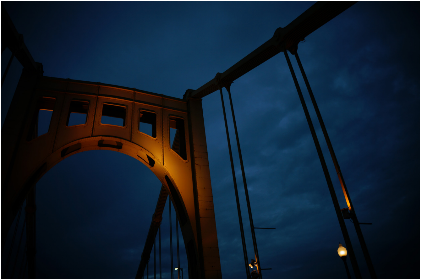
The Clemente Bridge: Pittsburgh, PA
